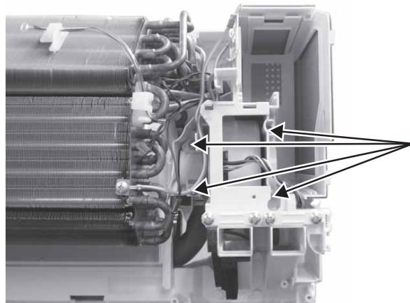
15. Remove the 4 screws holding the control board, then pull out the control board.
