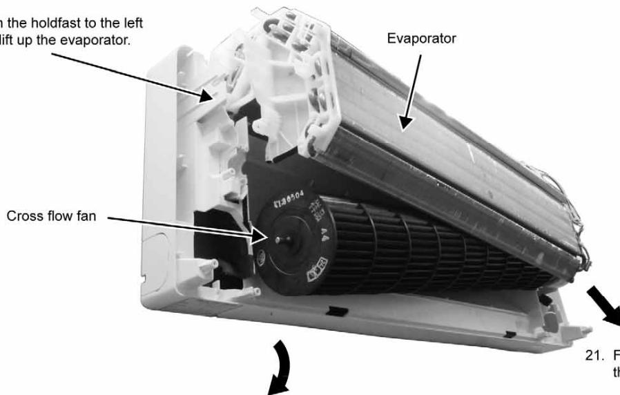
21. Fan motor can be removed after the removal of the cross flow fan.
